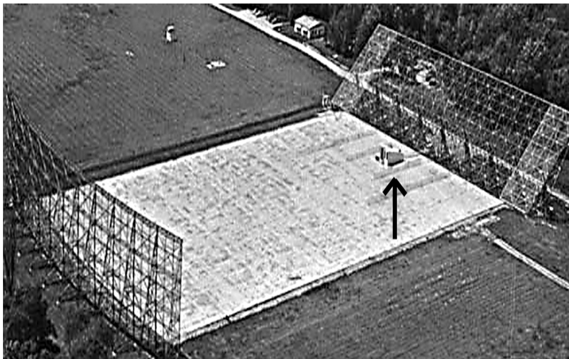
Figure 8.3: Schematic drawing of the Big Ear telescope. The arrow points to a pair of horns.
